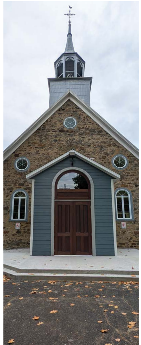
New concrete steps.
