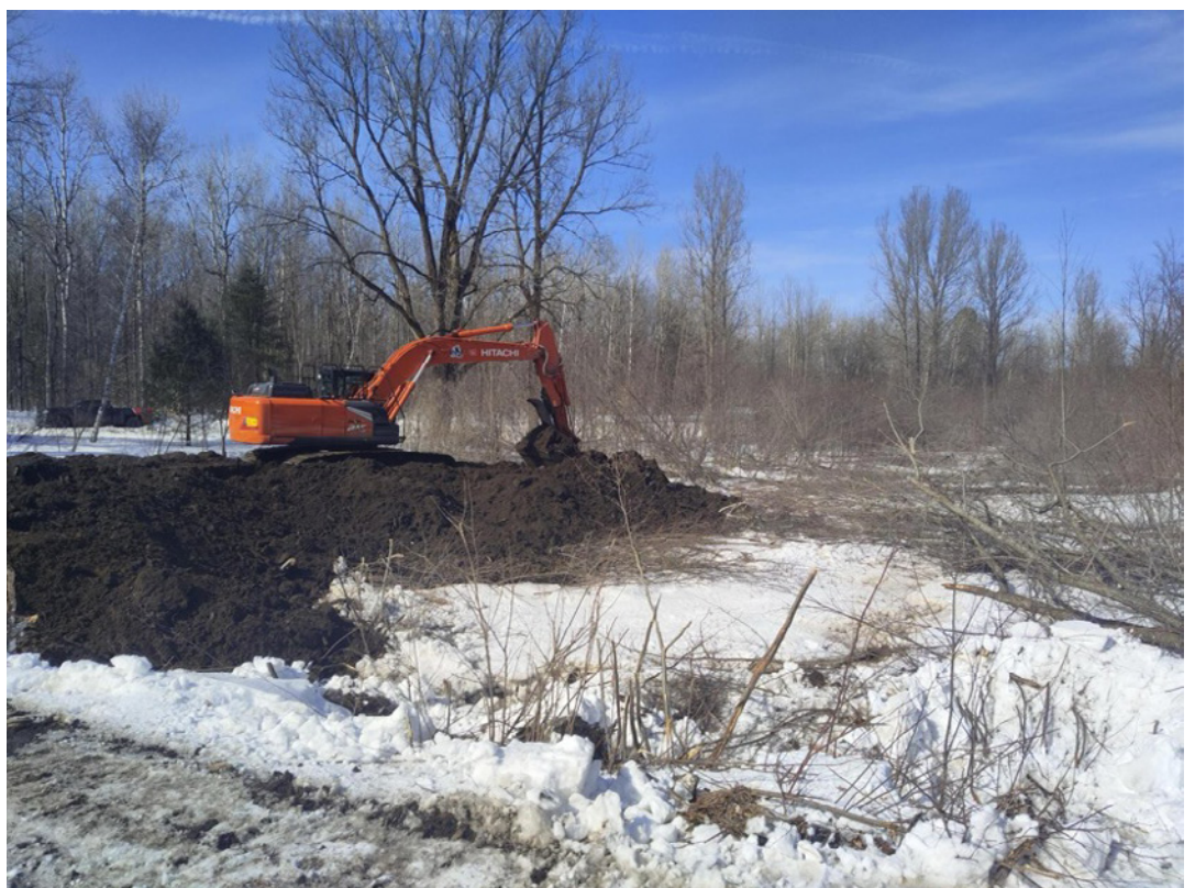
Ongoing progress at the Masta marsh.
