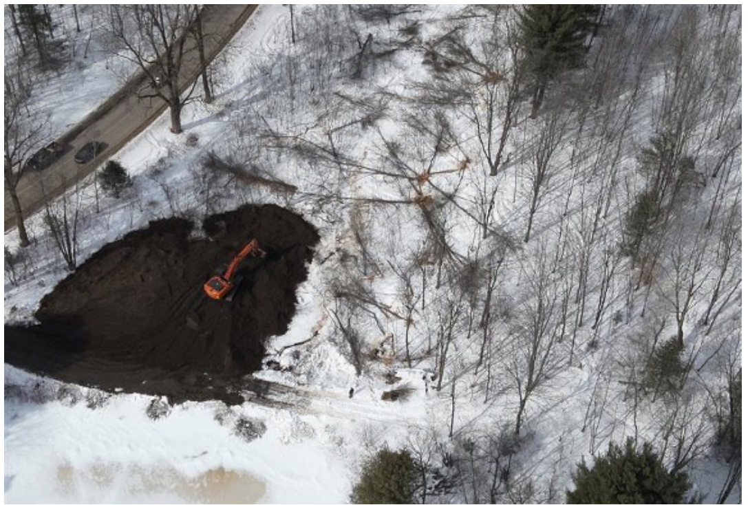
Aerial shot of the project's initial steps.
